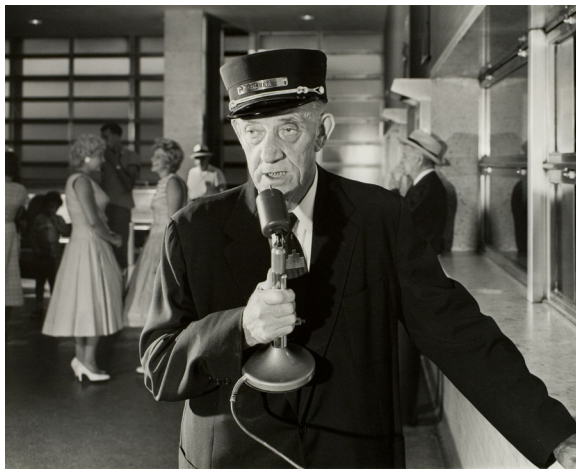
Buck Stewart Calling Trains at The Roanoke Station, 1956
