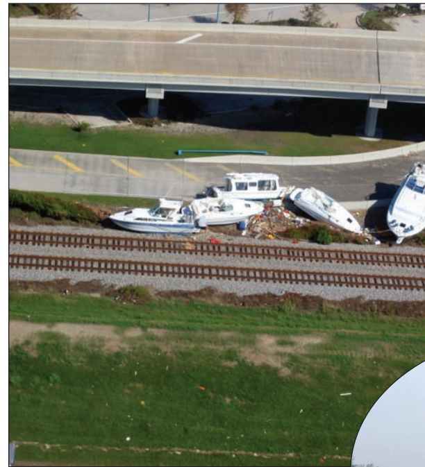
Flooding and wind littered NS' rights of way with debris.
