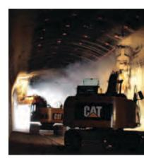
Contractors use an excavator, in top photo, to remove a boulder and other material while raising the elevation of the Cooper Tunnel. In middle photo, an Alpine roadheader mounted on a rail car grinds exposed rock inside the Hatfield Tunnel Main Two Track. At bottom, two excavators with roadheader attachments grind a notch in the concrete liner of Hemphill No. 1 Tunnel.
