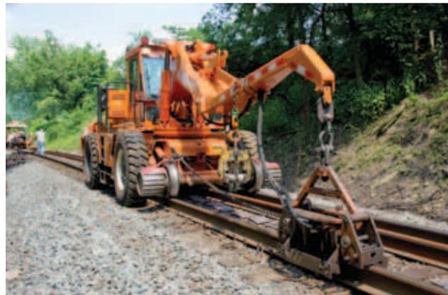
■ Top: **Josh Davidson**, a flashbutt welding machine operator on a welding gang based in Harrisburg, maneuvers the welding arm into place over two rail sections to be fused together. Davidson's gang set daily records for the number of rail welds, including 35 on one day. Typically, the daily goal is 15 welds.
