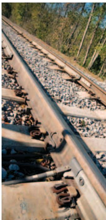
■ Wheel impact load detector, or WILD, sensors are installed on the rail and covered by a protective metal panel, shown above, at a WILD site in Ironton, Va.
