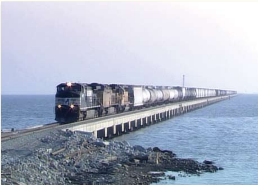
The first train moves across the Lake Pontchartrain trestle, restoring rail service to New Orleans just 16 days after Hurricane Katrina washed nearly five miles of track off the bridge into the lake. Norfolk Southern people repaired the bridge in record time, safely and under extremely challenging conditions.
