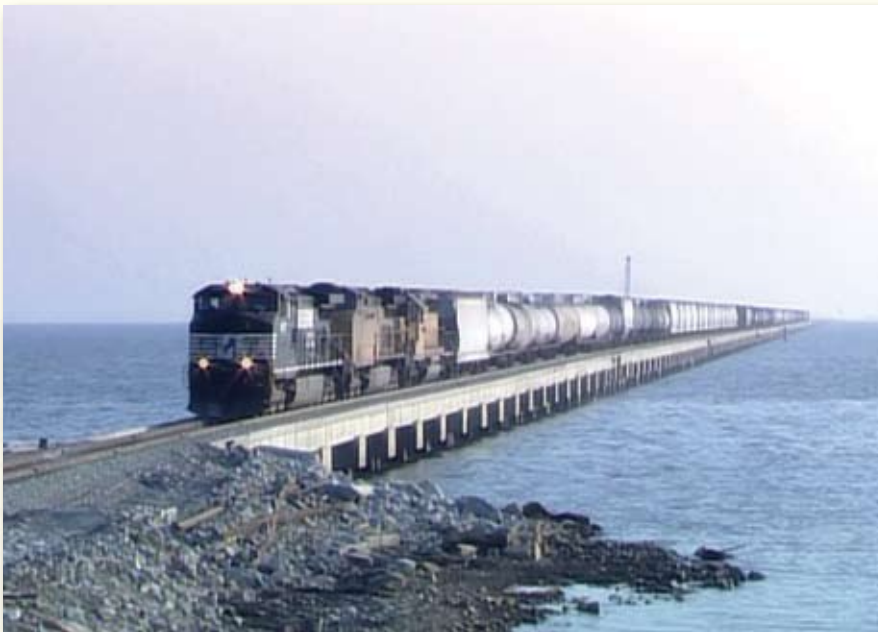
The first train moves across the Lake Pontchartrain trestle, restoring rail service to New Orleans just 16 days after Hurricane Katrina washed nearly five miles of track off the bridge into the lake. Norfolk Southern people repaired the bridge in record time, safely and under extremely challenging conditions.
