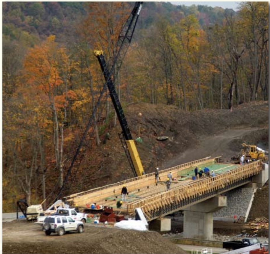
This railway bridge being constructed at Clarksburg, Pa., provides a more direct connection to the Keystone Generating Station, shown above left.
